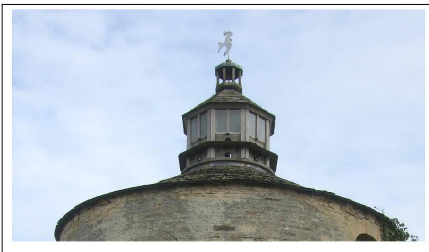
In 1998 the dovecote was fully restored. The entire roof structure was replaced, including the lantern top. A new weathervane in the shape of a red kite – reintroduced locally and now a common sight over the village – takes pride of place above the new lantern and can be glimpsed from West Street.
