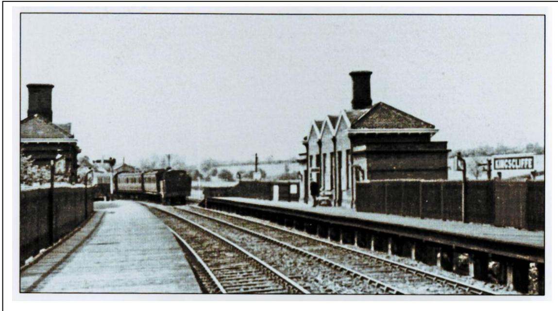
Goods traffic was always important at King's Cliffe station and a high-level dock was installed to allow goods to be loaded by tipping into railway trucks. The dock was extended and raised slightly in 1934 to accommodate more railway trucks.
